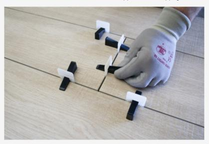
The placement of a locked joint greater than 25% is not recommended to avoid the appearance of uneven or lippage between adjacent pieces. Claims of material placed on a locked joint greater than 25% will not be accepted.
