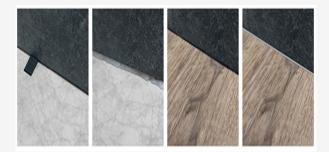
Lay the wall tiles at a height or 6 mm. Also place 10 mm perimeter gasket between wall and C&F. Fill the gap with silicone and place the board under the tile. Grout.
