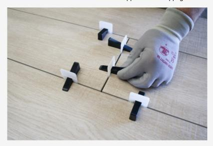
The placement of a locked joint greater than 25% is not recommended to avoid the appearance of uneven or lippage between adjacent pieces. Claims of material placed on a locked joint greater than 25% will not be accepted.
