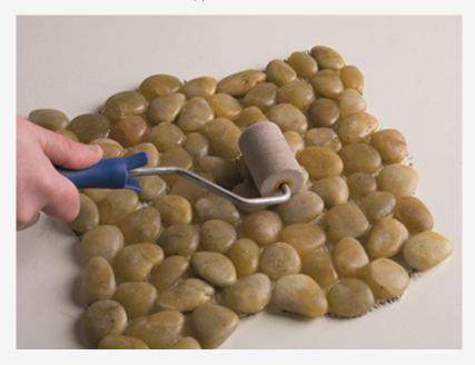
Important: Check the stones before installation, mix the sheets from different boxes to obtain a more homogeneous tone variation. For a better choice, get 5% additional quantity to the one needed.
