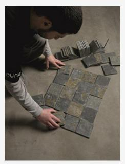
As we are dealing with natural materials, shade variation depends on the stone composition, which will be defined by the area of the quarry from which stone are extracted.
