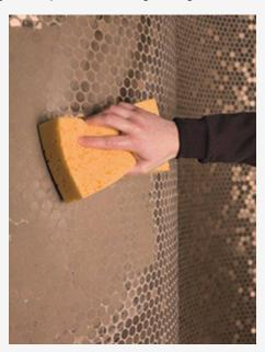
Use a damp sponge and clean water to wash off the excess of grouting paste from the surface. It is very important to do this before the paste dries. If this happens, use a cement remover to clean the surface. (not apt for stone)
