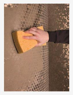
Use a damp sponge and clean water to wash off the excess of grouting paste from the surface. It is very important to do this before the paste dries. If this happens, use a cement remover to clean the surface.(not apt for stone)
