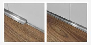
Leave 10 mm. expansion joint, fill with silicone and cover with a scotch molding.
