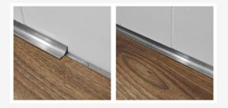
Leave 10 mm. expansion joint, fill with silicone and cover with a scotch molding.
